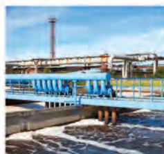
Waste Water Treatment Plant
